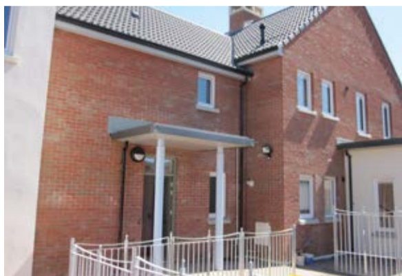
Building our new Short Break Service in north Belfast
